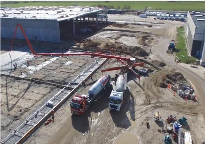
Due to heavy steel fiber reinforcement using 1700 N/mm<sup>2</sup> high strength steel fibers at a dosage rate of 50 kgs/m<sup>3</sup> (85 lbs/cu yd) and our proprietary anti-shrinkage additives, our composite concrete is much stronger. Therefore we were able to provide a much thinner slab thickness exceeding defined loadbearing demands. Our solution was 350 mm slab (13 in) with 540 mm (21 in) perimeter beams.
