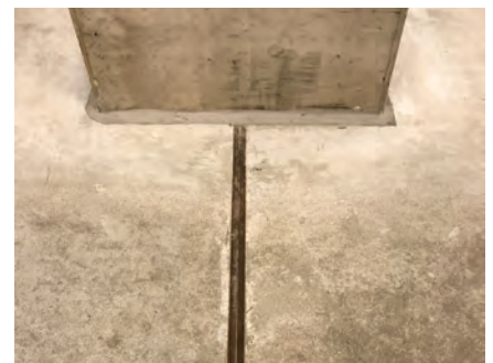
Figure 1c: A Primekss construction and column isolation joint at seven years of age.
