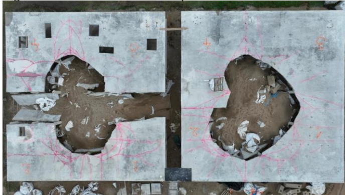
Fig.4. Failure pattern for (left) – SFRC, (right) - SFRSSC.
