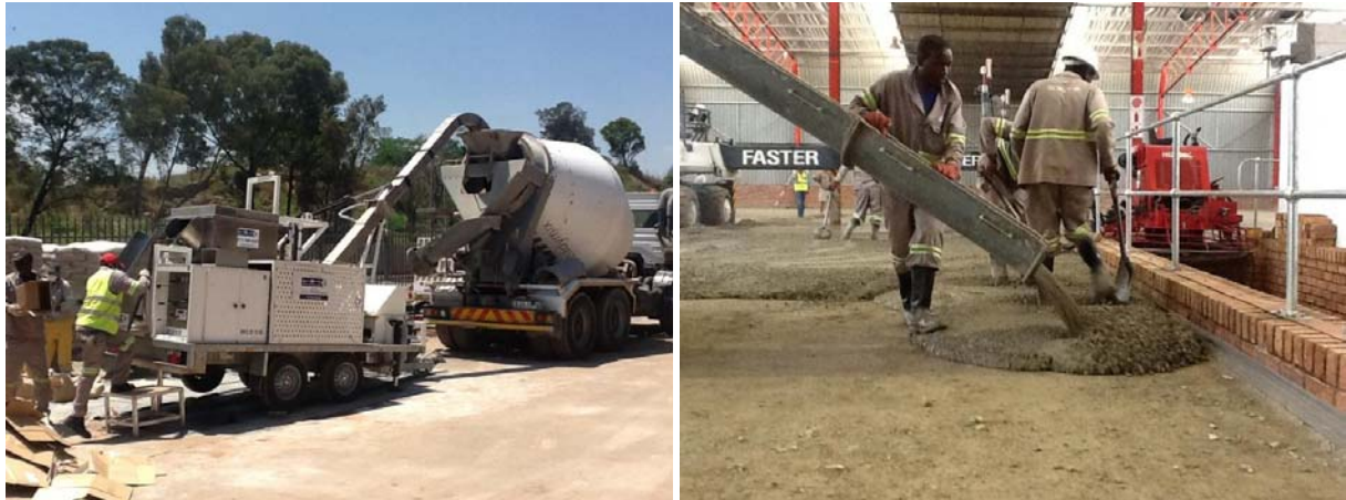
Figure 2: Addition of the PrimeDC, PrimeFlow additives and steel fibres to a specially designed concrete mix on site for the Prolecon Project in Johannesburg, South Africa.
