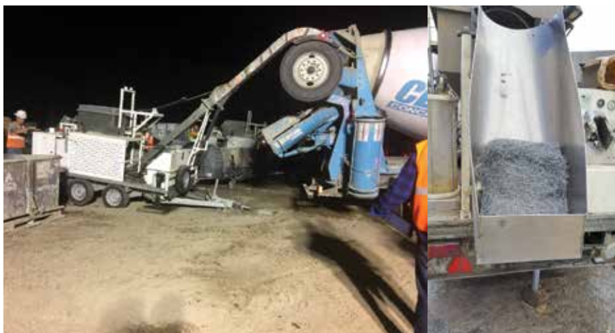
Fig. 1: Fiber blower in action at a Gresser Companies, Inc. building site in Minneapolis, MN (left) and chute with loaded fibers (right)
